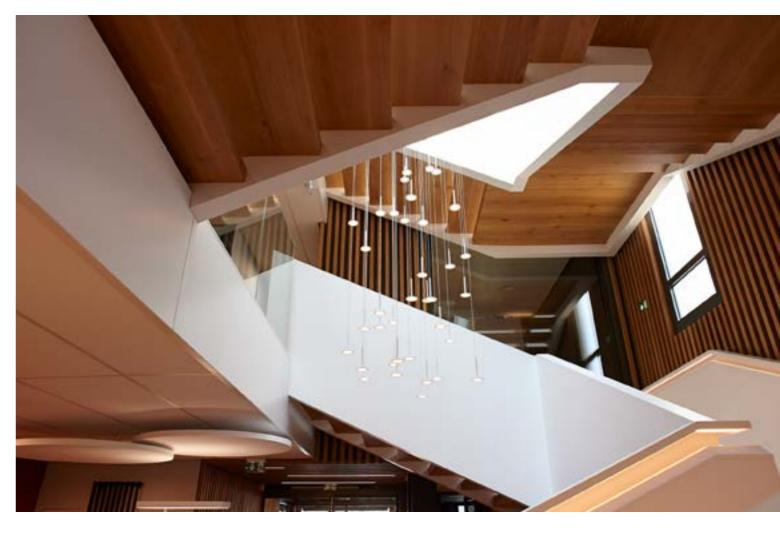
A handrail and subtle lighting in one: the delicate LED strip was concealed in the pre-milled groove.
